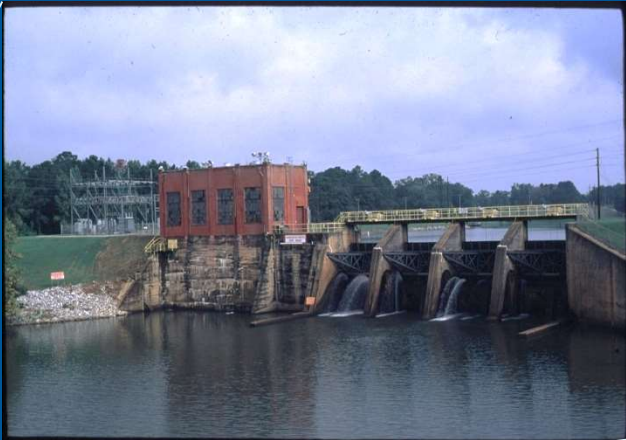
Gantt Hydroelectric Plant
